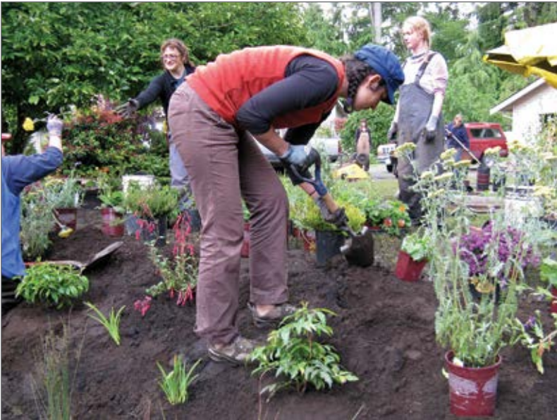
Rain garden construction (Photo: Kim Gridley)
