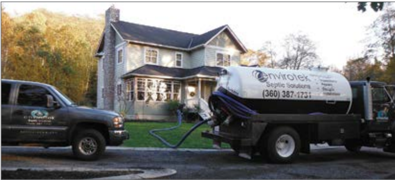
Septic system pump truck (Photo: Alan Chapin)
