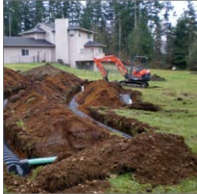
Drainfield installation (Photos: Alan Chapin)
